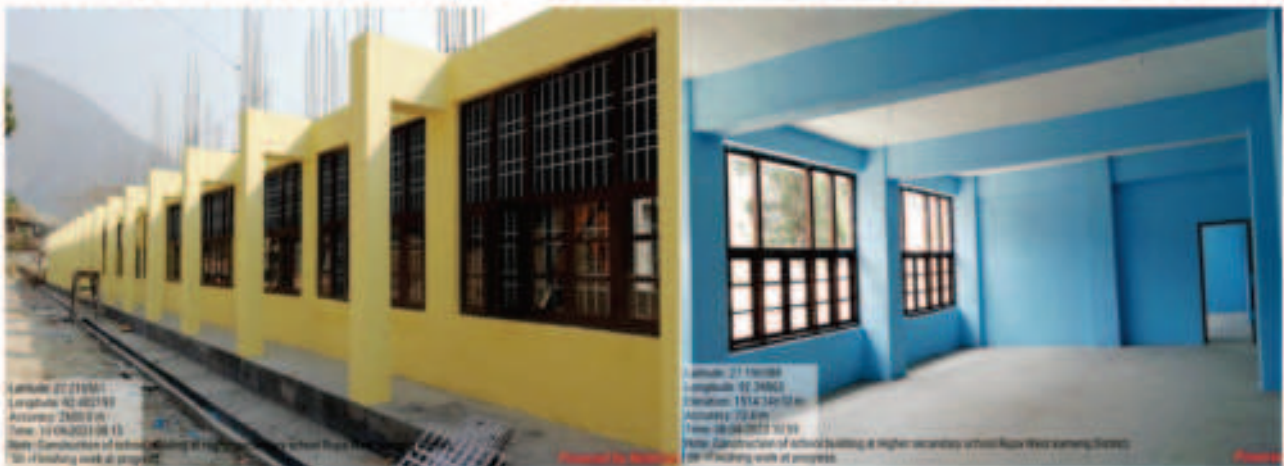
Name of Work: - Construction of School building at Higher Secondary School Rupa, West Kameng District, AP.
