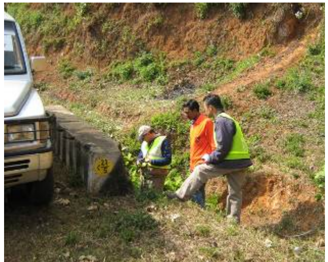
Culvert Detailing and Inspection, Umsning, Meghalaya
