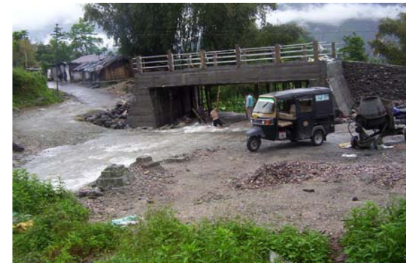
Minor bridge in progress
