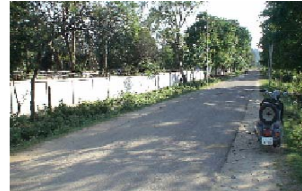
Boundary wall, General Hospital
