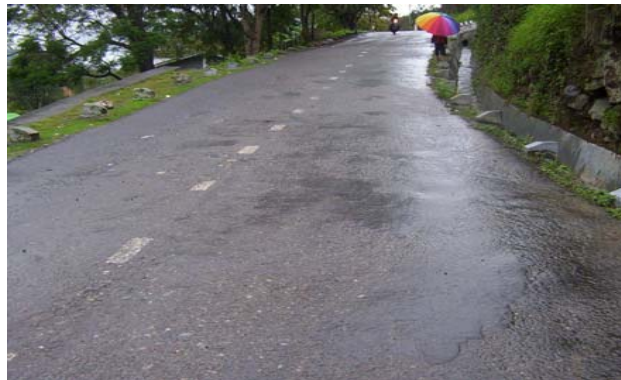
Blacktopped road with side drains
