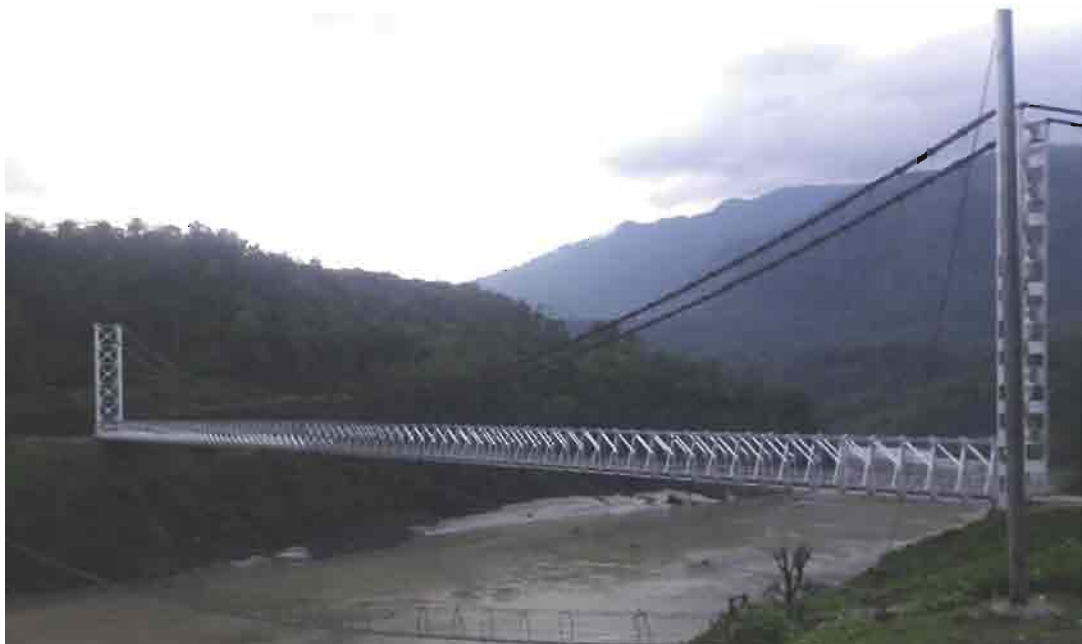
Steel suspension bridge over river Siang at Kodak in Upper Siang District under NLCPR (Span-210 m)
