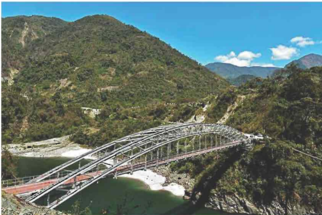
Steel Arch Bridge over Lohit river under NLCPR (Span-135 m)
