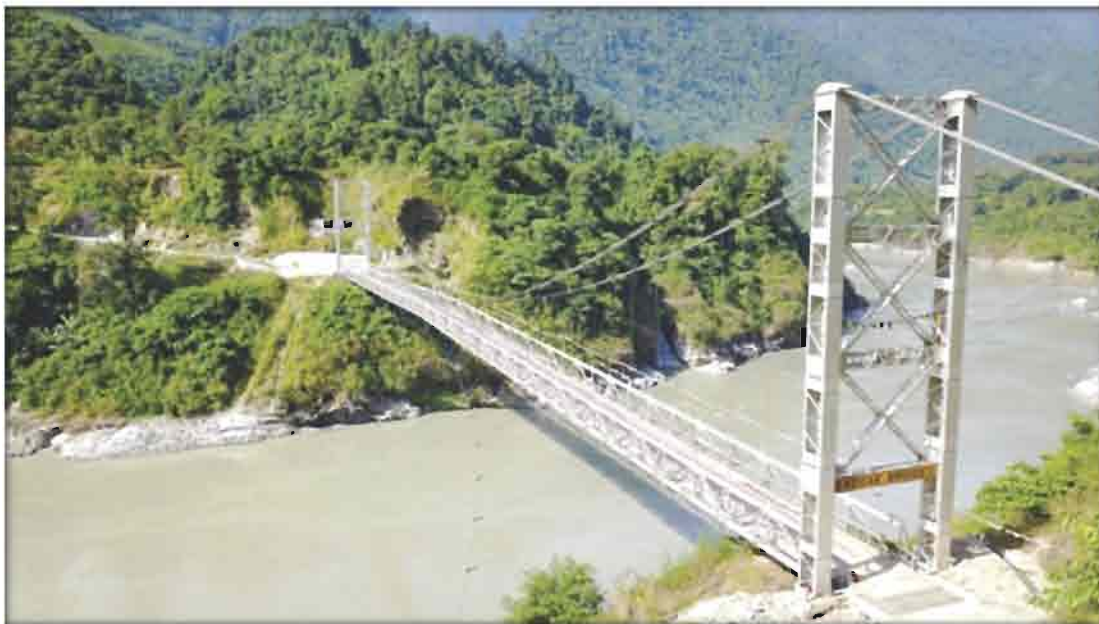
Steel suspension bridge over river Siang at Kodak in Upper Siang District under NLCPR (Span-210 m)
