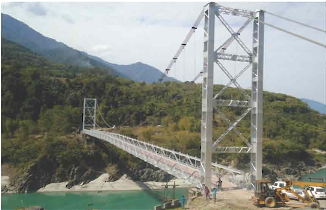
Steel suspension bridge over river Siang at Nubo in Upper Siang District under RIDF (Span-218.50 m)
