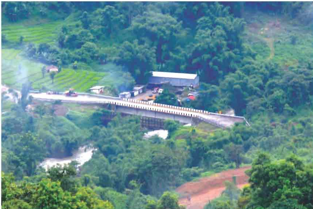
Longding - Nokajan Road (RCC Bridge over Tissing river.) under NEC (Span-40 m)
