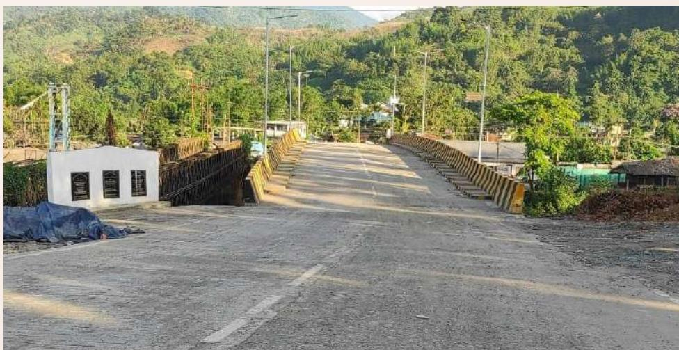
DOUBLE LANE COMPOSITE STEEL GIRDER BRIDGE (Span 60 mtr)
