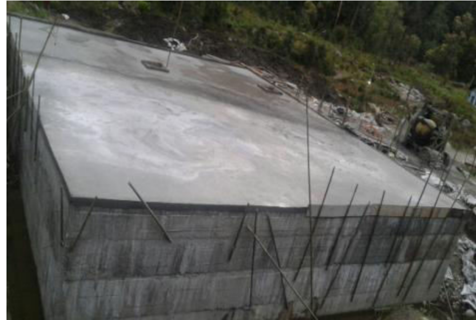
ANCHOR BLOCK RIGHT BANK
