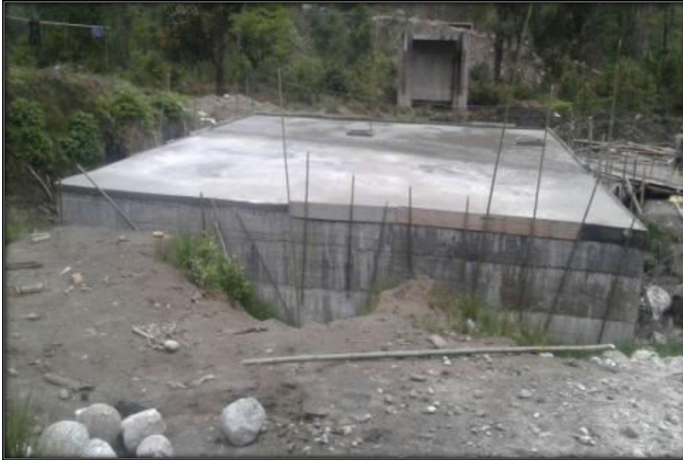
ANCHOR BLOCK RIGHT BANK
