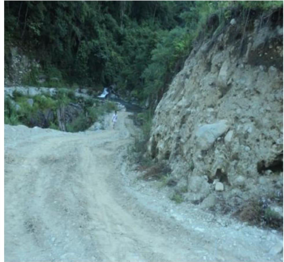
FORMATION CUTTING AT CH: 11.60KM
