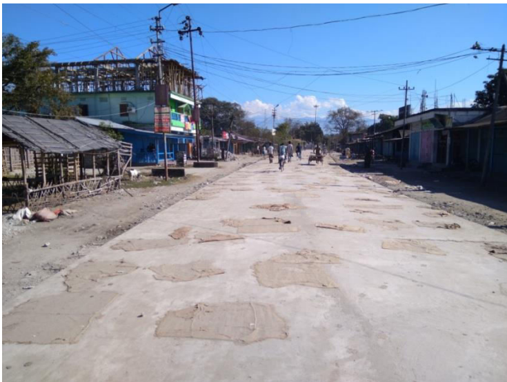
Construction of C.C. Road in Tezu Township
